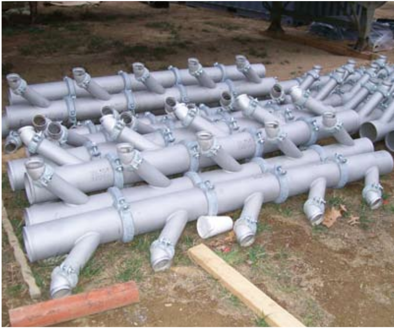
Pre-assembled, mechanically joined wye fittings awaiting installation above cell chases.
