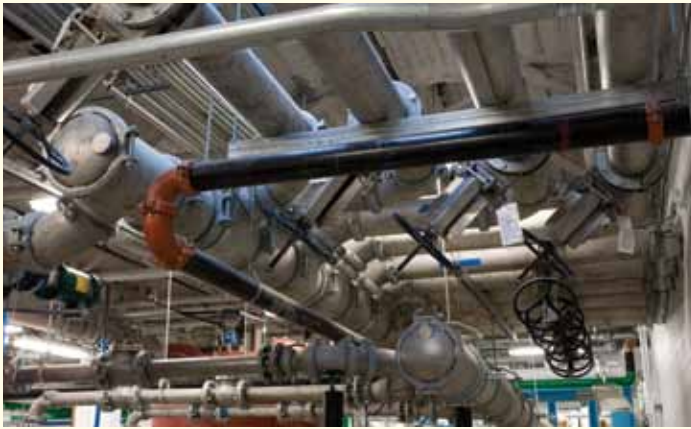
Waste Piping Can Be Routed Over-head, Horizontally
