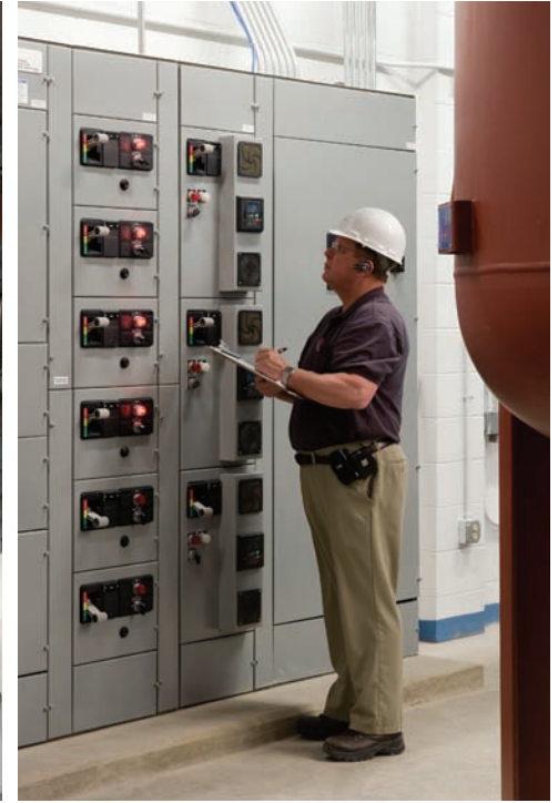
Vacuum system motor control center
