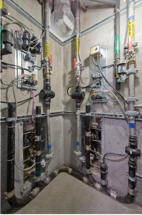
Vacuum drainage system chase
