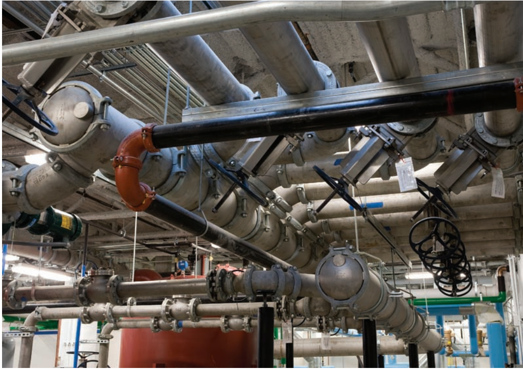
Overhead vacuum drainage system piping
