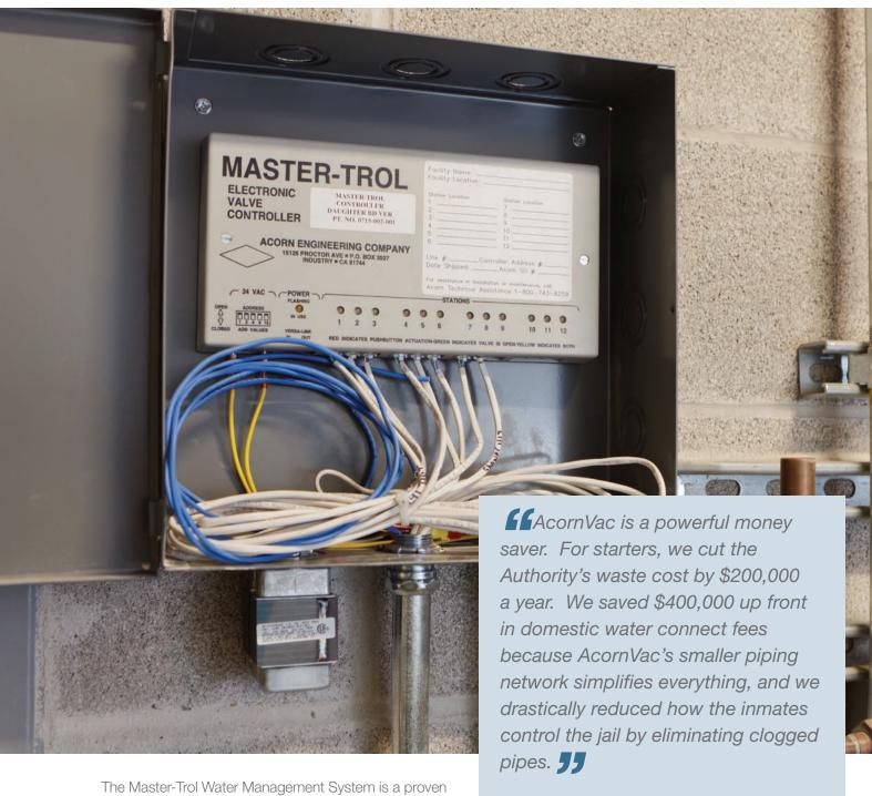
The Master-Irol Water Management System is a proven tool in reducing inmate water usage; it limits use of plumbing fixtures and improves the sustainability of a facility. Master-Trol limits the number of flushes and monitors water usage by reports, graphs and charts, allowing for calculated water savings. This ultimately leads to a reduction in overall water usage in correctional facilities and savings in utility costs.
