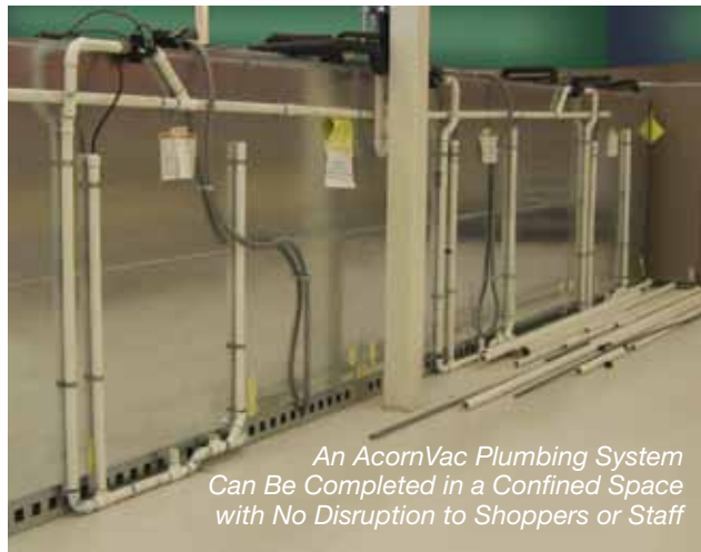
Back view of a vacuum plumbing system installation on a refrigerated case
