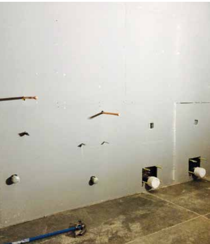
Bathroom drywall finish with carriers for toilets
