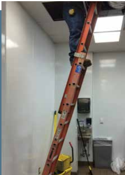
The ceiling space in the kitchen where the vacuum system is located
