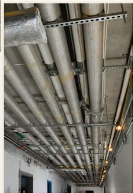
Figure 2 Overhead vacuum waste piping
