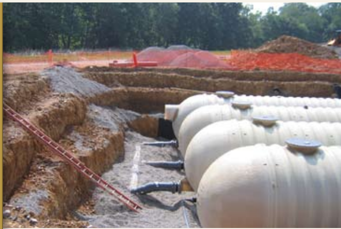
Figure 6 Underground storm water storage tanks
