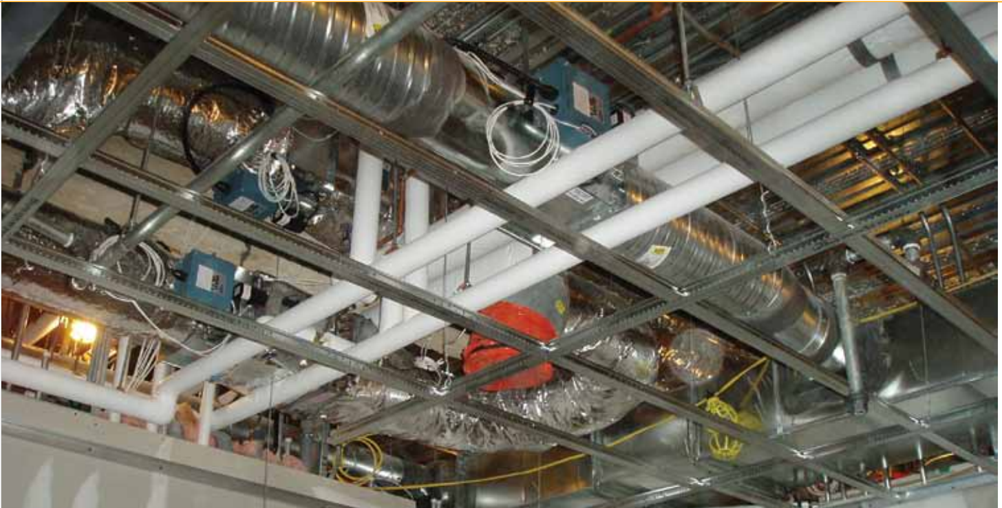
The use of a vacuum plumbing system eliminated the need for any floor excavations, a critical construction element given the highly volatile conditions in the lab.
