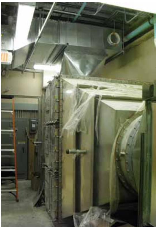
The HEPA-filtered central exhaust system plays a key role in maintaining the integrity of the space by filtering out all lab exhaust prior to discharge into the atmosphere.
