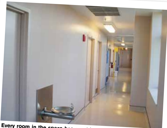
Every room in the space has an airlock. Pressure indicators are located above each door so occupants can continuously monitor room pressures.
