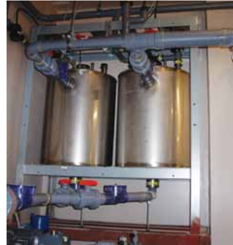
Left: In the BSL-3 lab, researchers conduct experiments on contagious materials in gas-tight enclosures, thus the need for a fail-proof wastewater system. Right: The two 60-gallon vacuum system tanks collect wastewater 8 feet above the ground.
